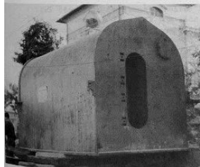
Steel Gothic type Shelter on road side at CIVITAVECCHIA as used in the above position
